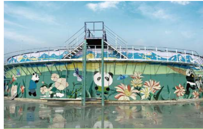
Municipal Sewage Treatment Project
