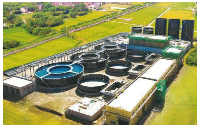
Dairy Wastewater Treatment Project
