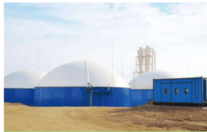
Inner Mongolia Biogas Project
