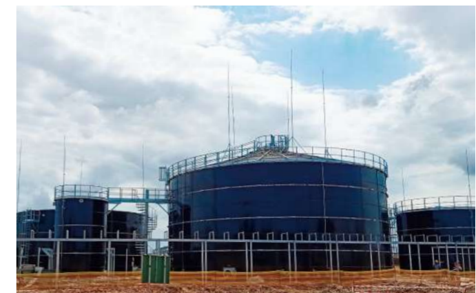
AB InBev WWTP Project in Mozambique
