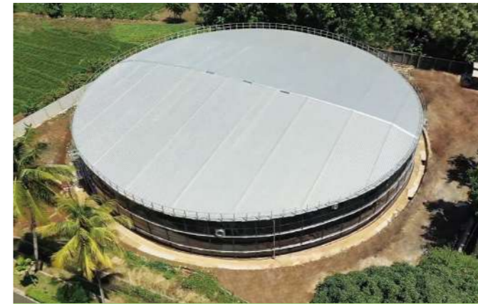
Potable Water Storage GFS tanks
